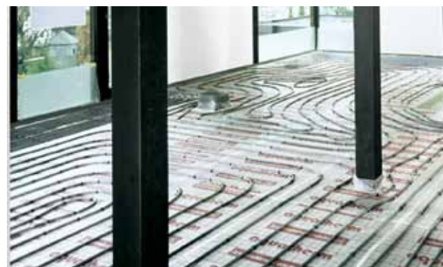
Underfloor heating installation
